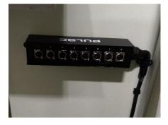
The stage box is fixed to the wall at the side of the stage on the right hand side, looking from the hall. Channels 3,4 and 5 are connected to channels 3,4 and 5 of the main mixing console in the audio cabinet.
