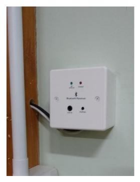
The audio system is connected to a Bluetooth connection box in the rear corner of the stage. close to the audio cabinet. Output is via channel ST2.
